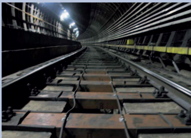
Fig. 7: FFU on heavy mass spring system – metro Vienna – koocoo
