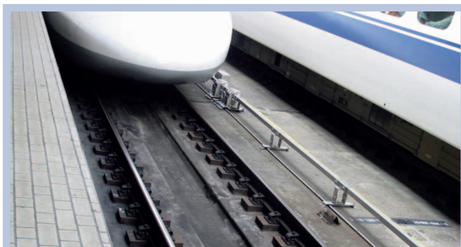
Fig. 1: FFU twin block sleepers in Shinkansen station – Japan – SEKISUI
