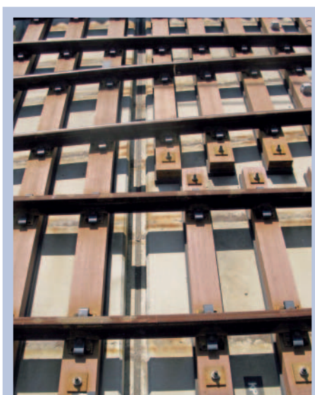
Fig 4: FFU sleepers on the regional track Osaka – Horoshima – koocoo
