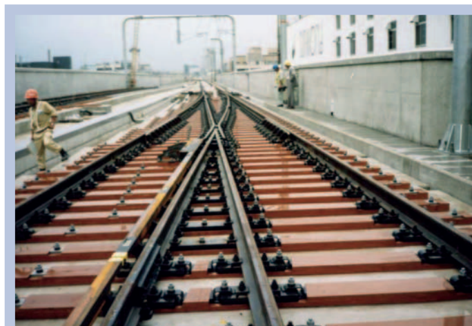
Fig 3: switch on FFU in slab track – Japan – SEKISUI
